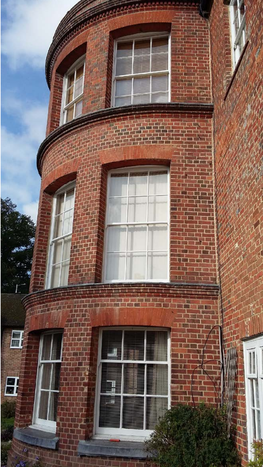
North Elevation (to front driveway)
